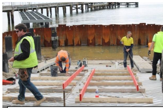
This is how you lay concrete under water
